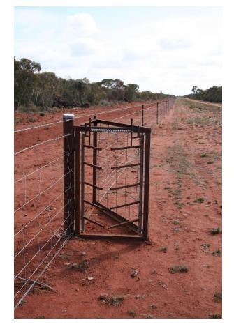
Figure 1. Goat fence and one-way gate.
